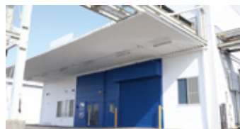
AMC Nagoya: Mass production & testing
