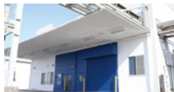
AMC Nagoya: Mass production & testing
